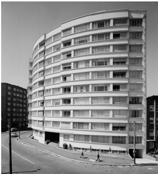
Figure 1 Bolot's Wylde Street Cooperative flats (1947–1950). (Source: Max Dupain, courtesy of the Australian Institute of Architects)
